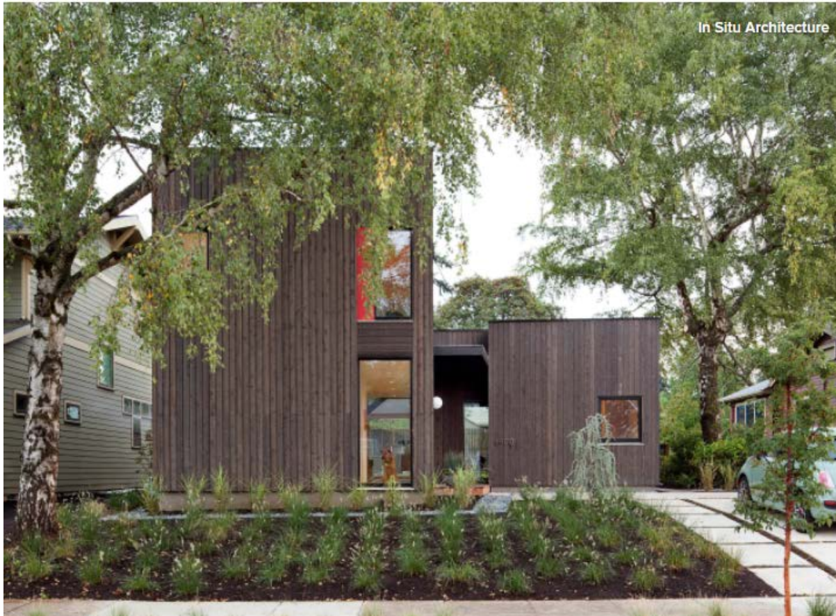
Passivhaus in Portland (Oregon), USA
